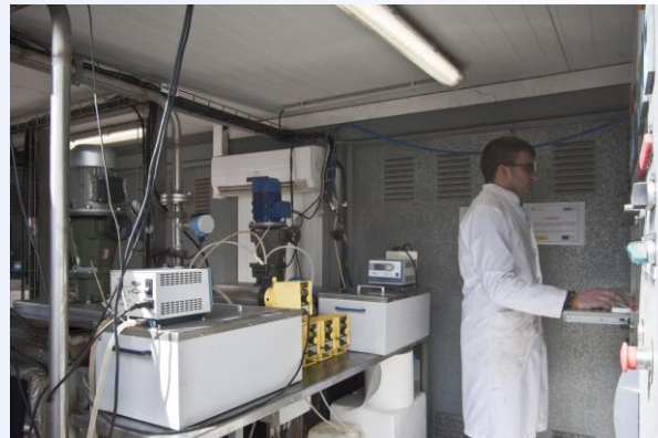
Pilot plant Panamox® process
